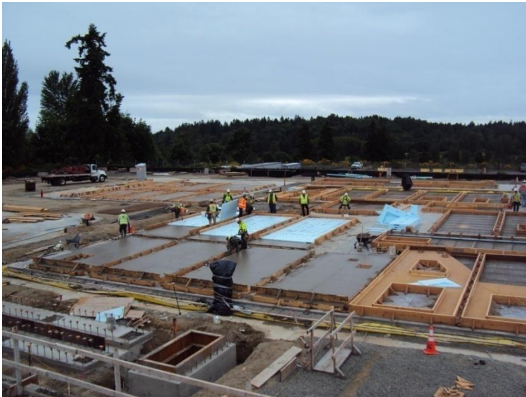
BMF Bldg. – Tilt Panel Forming & Casting
